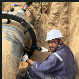
Pipe Cold Cutting
